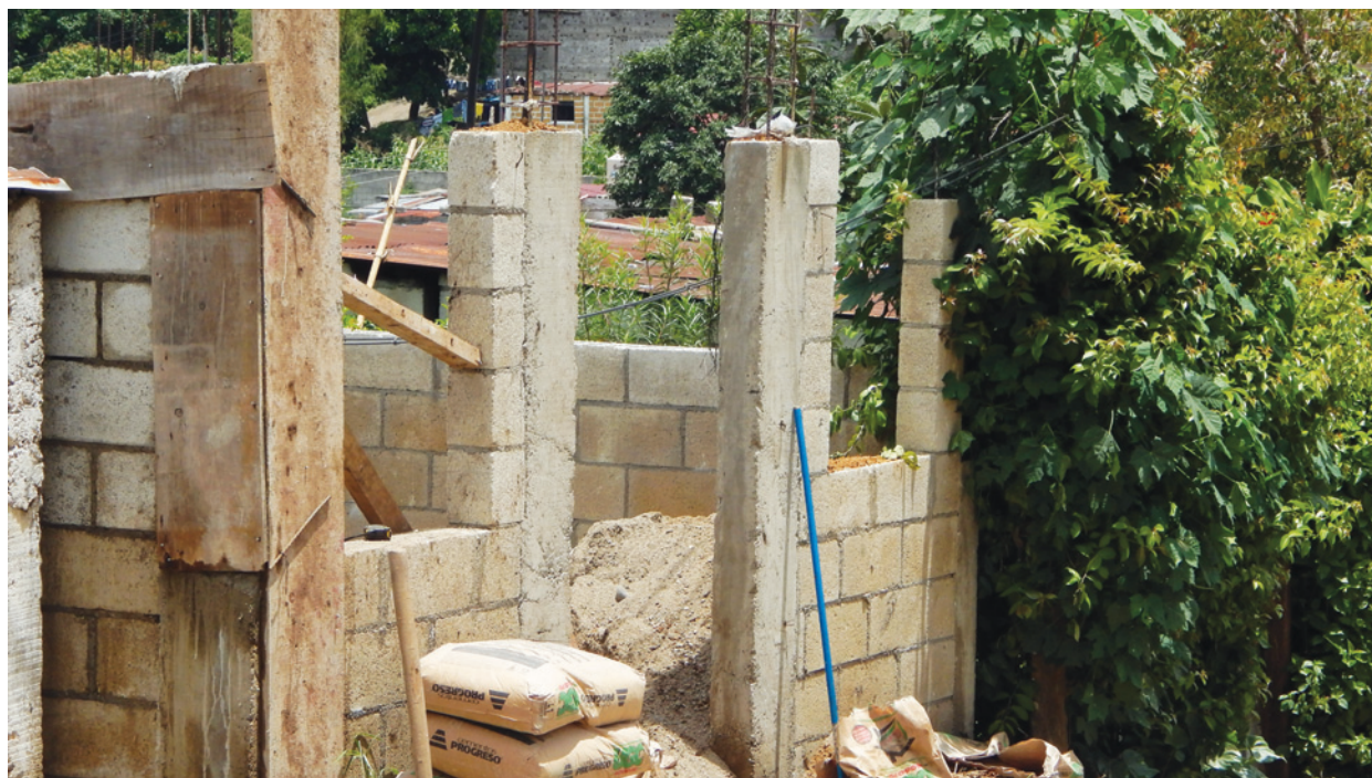
A new house for Blanca and Alexis starts to take shape.
